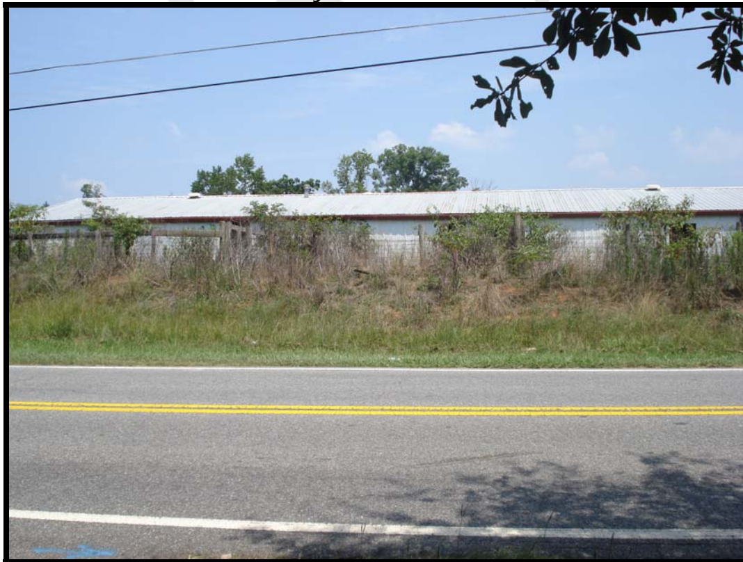
View Across the Street from Subject Site
